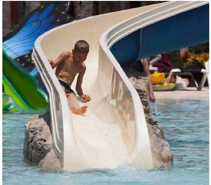
This slide exit is almost too vertical. A participant coming down head first could hit the concrete bottom.
